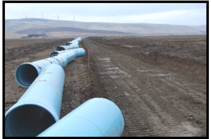
Gardena Farms Irrigation District #13's south lateral under construction. Pipe was stationed and ready for installation beginning in mid-January 2010.
