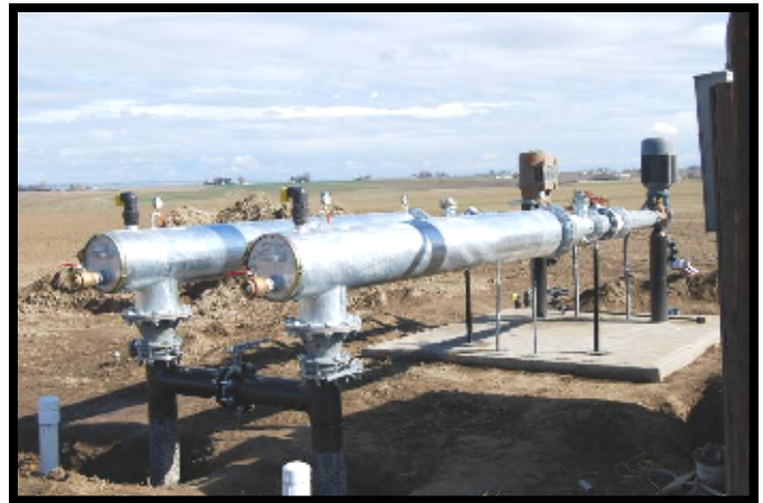
GFID #13 pumping station #19 near completion in mid-March.
